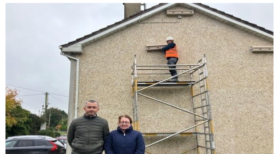
Installation of Swift Nest Boxes at Thomastown Area Office
