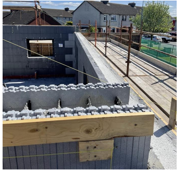
Construction of 2 Wheelchair Accessible Houses at the Old Community Center in Loughboy, Kilkenny The Houses are being constructed using Insulated Concrete Form (ICF)
