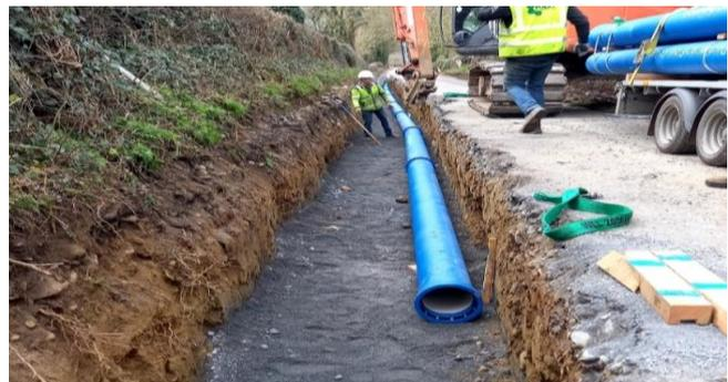
*Construction of Ductile Iron Rising Main to Rathduff Reservoir*
