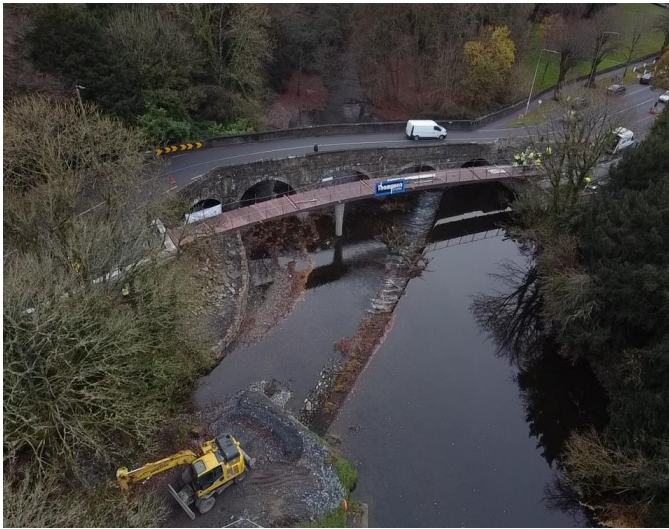
Drone view of new Footbridge & Existing Road Bridge.
