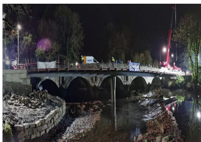
Photos of Bridge Transportation and installation on night of 23 rd November 2021
