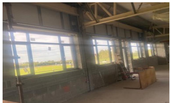
Installation of windows at Gowran Community Complex
