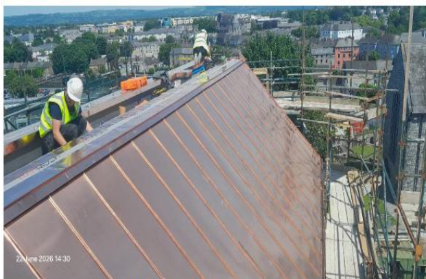
Copper roof cladding on rear annex
