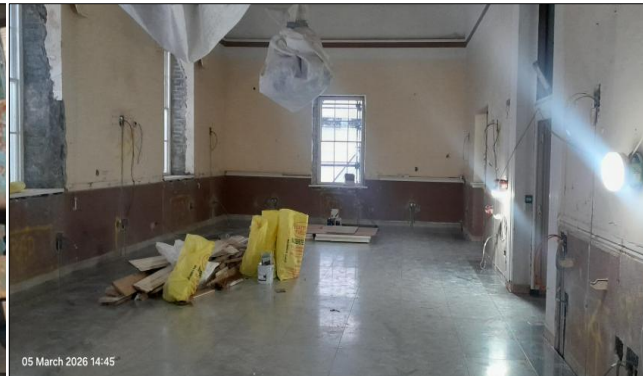
Installed raised access floor and traditional timber sash windows in Council Chamber
