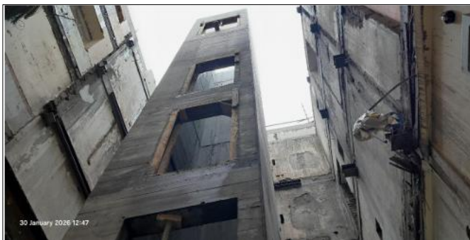
Boardmarked concrete lift- shaft to 4 th Floor
