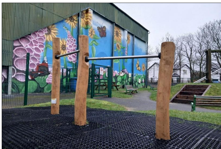
Mullinavat Playground- Installation of new somersault bars and soft-surfacing
