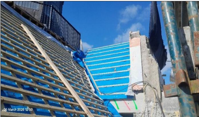
New pitch road to rear replacing old flat road (Returning building back to original profile)
