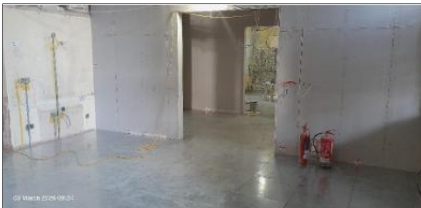
Installed raised access floor and slabbed partition looking from Mayors Parlour into Looby
