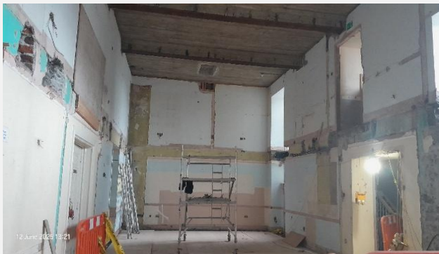
Second Floor: Mezzanine floor introduction removed allowing for reintroduction of window opens into
