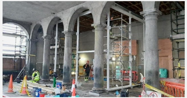
steel frame for glass reception area within Loggia
