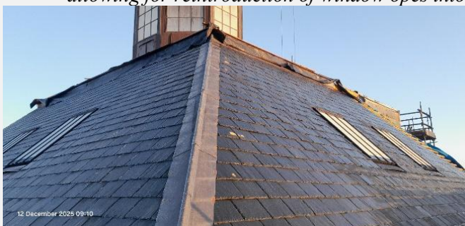
Roof Level: Re-slating of roof and installation of to rear
