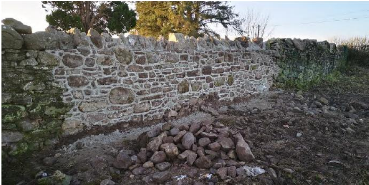
Community Monuments Fund repair works at Kilbeacon Graveyard 2025
