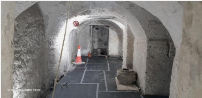
Basement - Restored walls, ceiling and floor and
