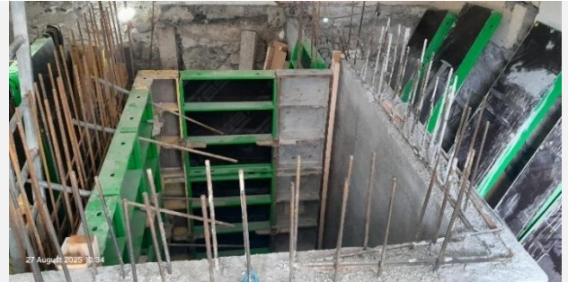
construction of lift shaft & stairwell in rear annex
