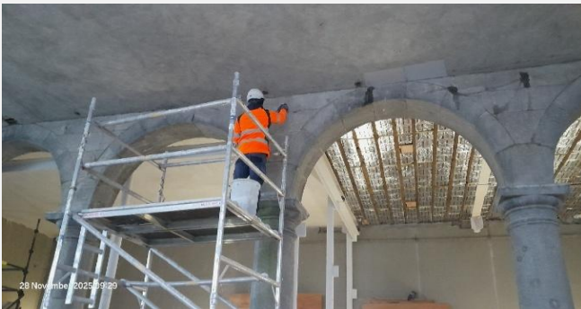
First Floor – Stone repair works and installation of
