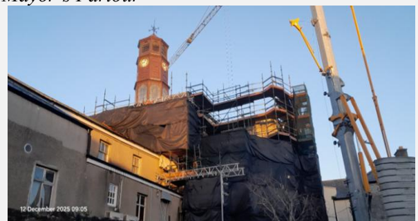
heritage roof lights & removal of 20 th Century flat roof annex.
