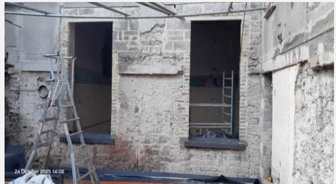
returning space back to double height ceilings and Mayor's Parlour
