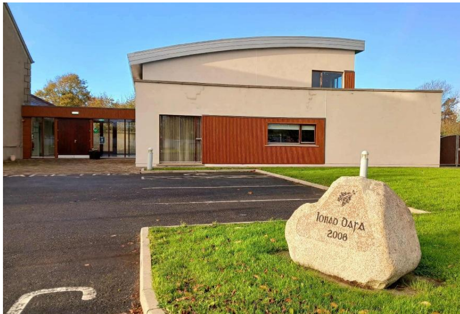
Cladding works carried out to Ionad Dara, Community Hall, Goresbridge funded under the Local Enhancement Programme 2025
