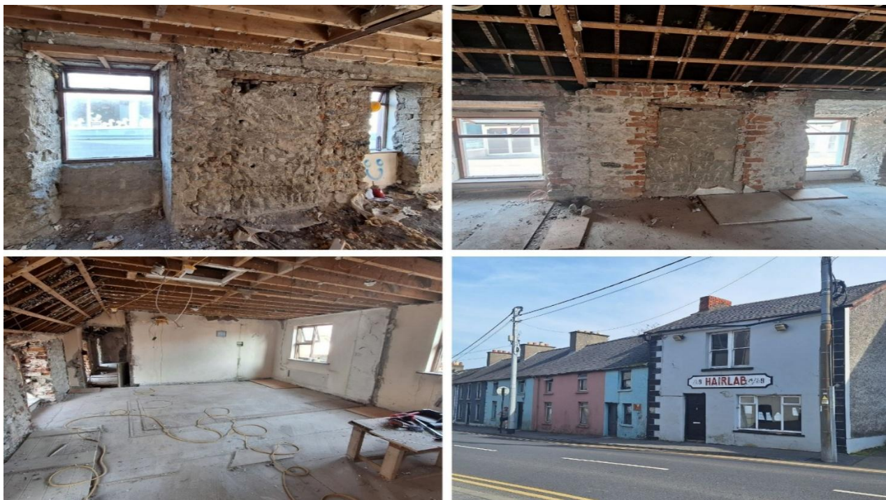
Commencement of construction works at property located at 6-9 Upper Patrick Street, Kilkenny City
