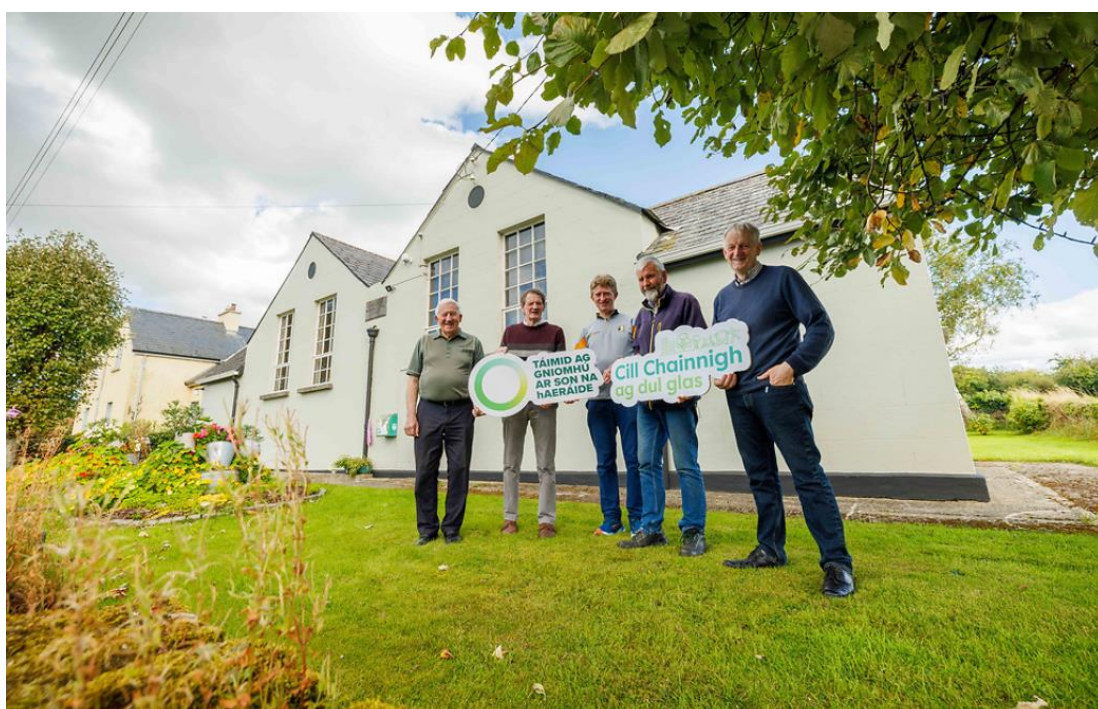
Tullahought Community Development are making the Community Hall more energy efficient and comfortable by insulating the roof and upgrading the windows. They are also installing a new composter for use in their fantastic flower displays.
