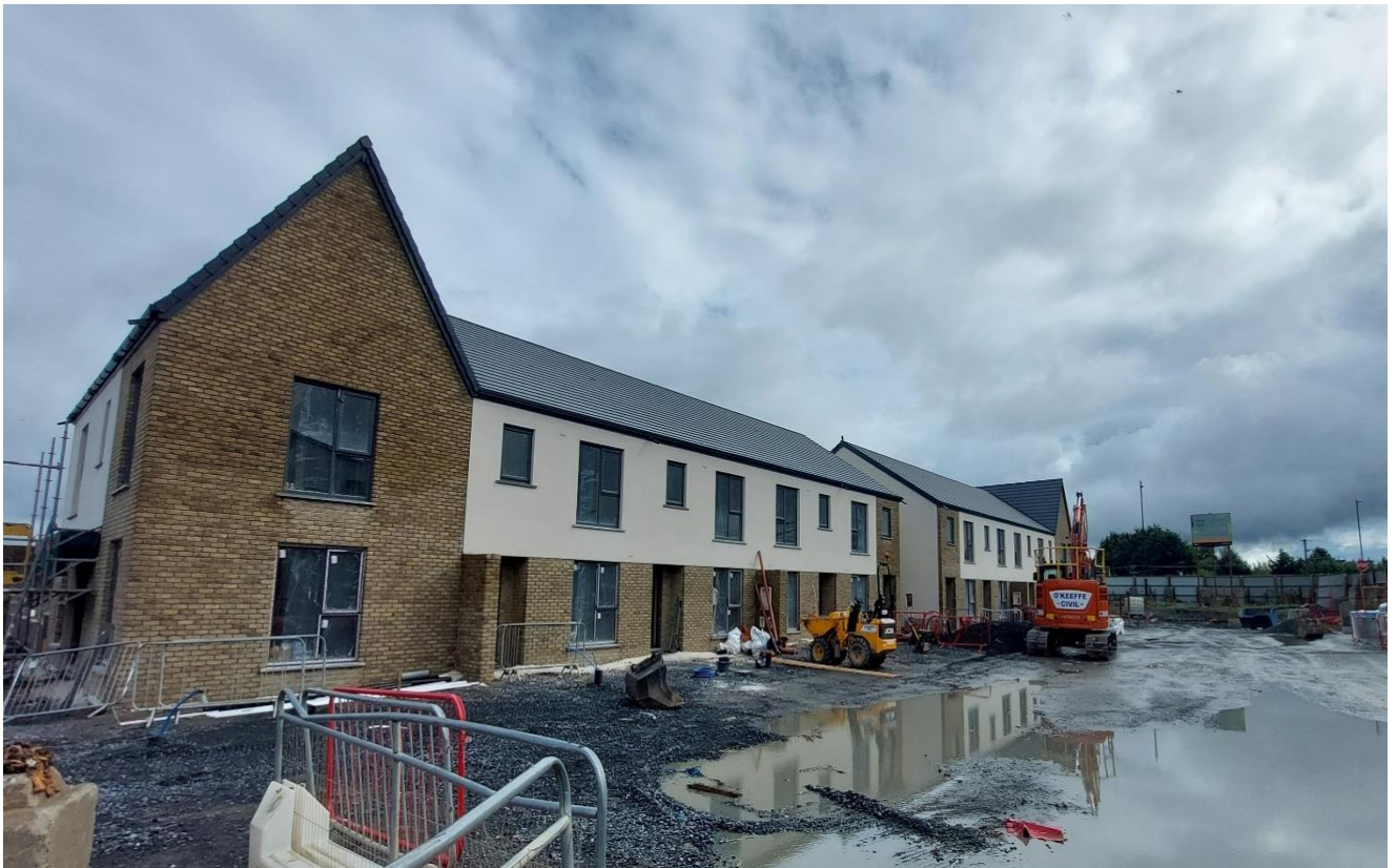
Part V units at College Park Crescent, under construction
