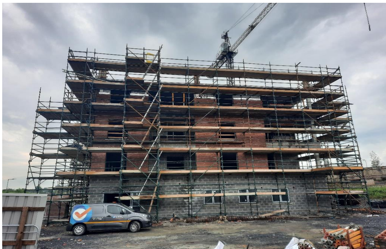
30 apartments at Castleoaks, Breagh Valley, under construction
