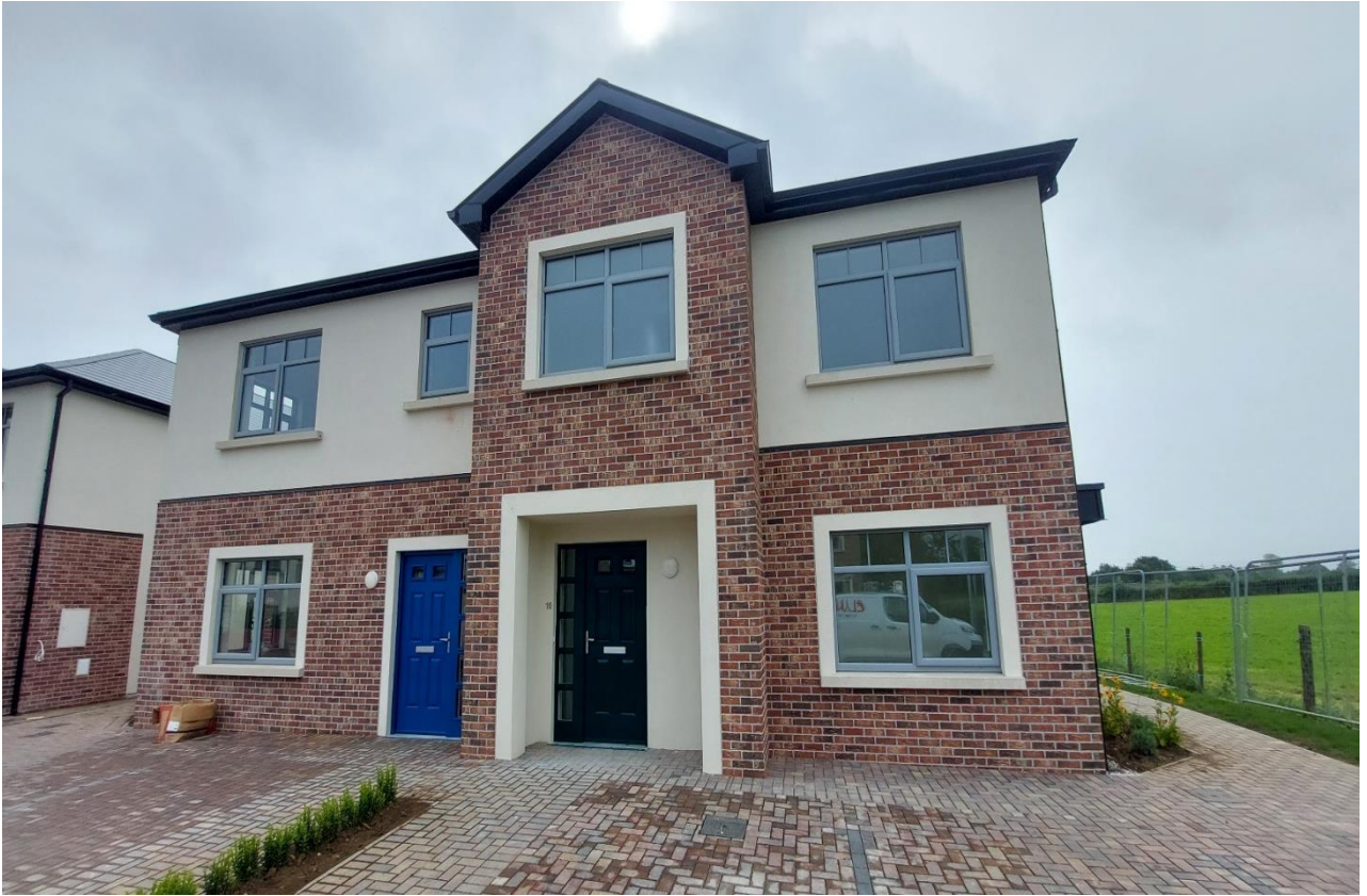
8 completed apartments at Foxmeadow, Loughmacask
