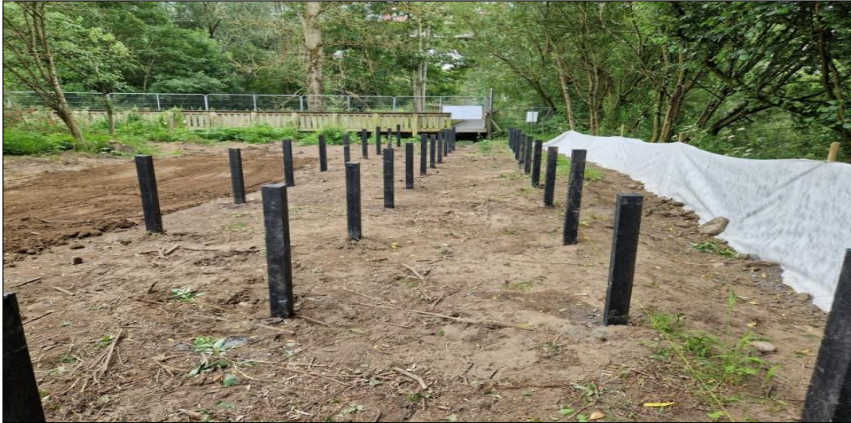
Phase One – Image of Pile Installation
