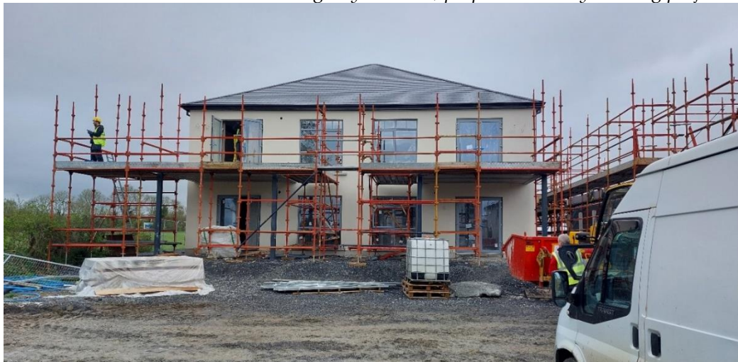
8 x 2 bed Part V apartments under construction at Fox Meadow, Kilkenny
