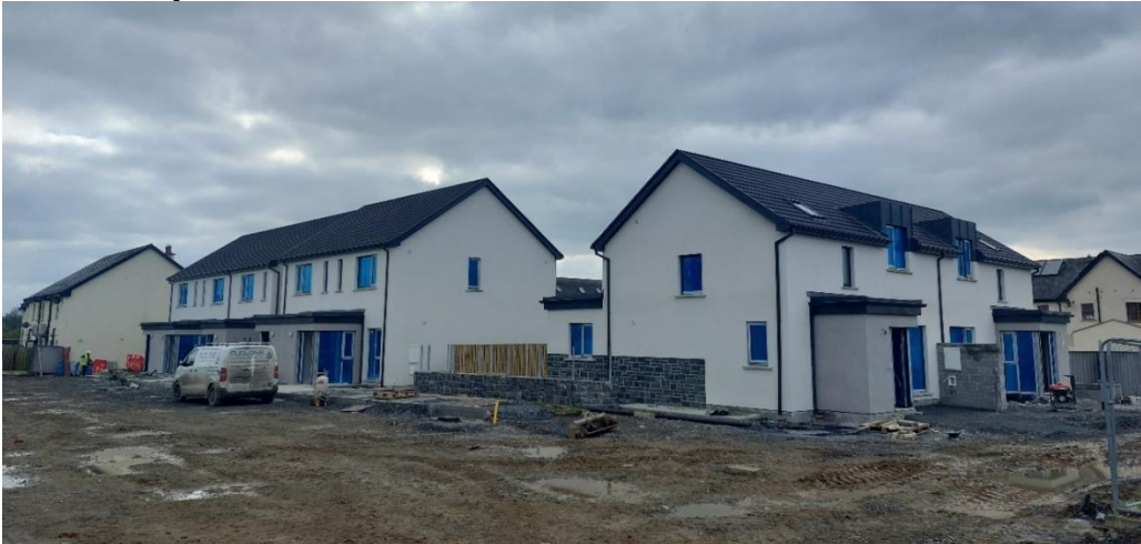
17 houses under Construction at Ogenty Gowran, proposed turnkey housing project
