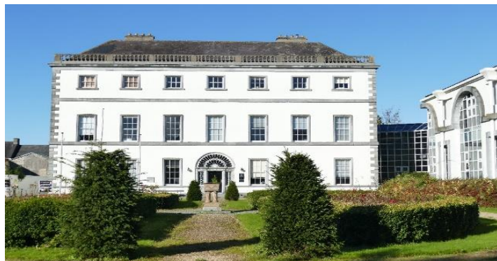
County Hall is one of the Council's top five energy using buildings in its portfolio
