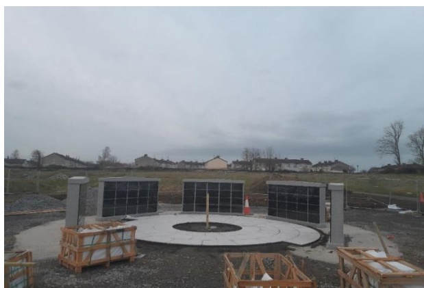
Progress to date on Columbarium Wall Garden St. Kieran's Cemetery
