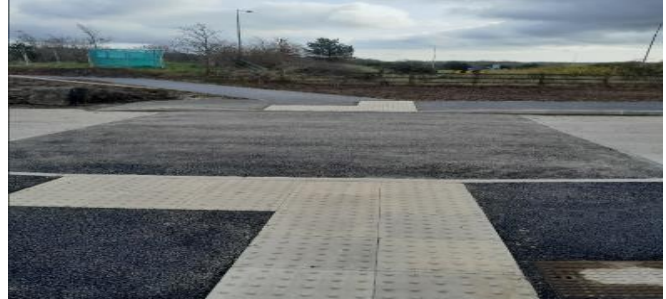
New Raised Uncontrolled Crossing Point to Park
