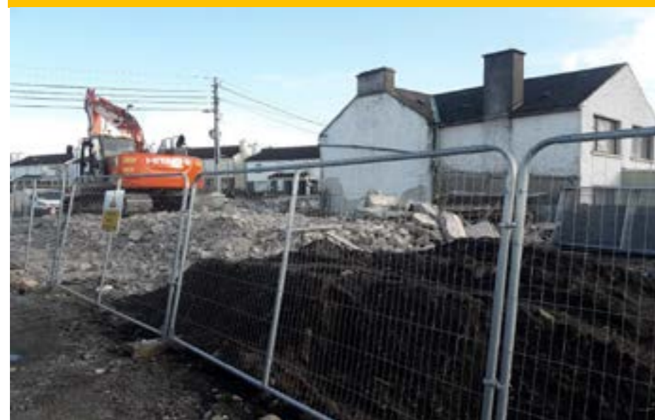
Demolition Works at Golf Links Road Site, Kilkenny City
