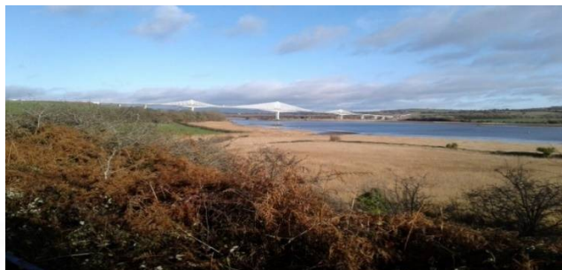
View of the recently opened Rose Fitzgerald Kennedy Bridge from the old railway line at Carrickcloney.
