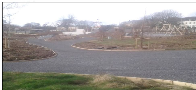
The recently installed playground pieces in Ferrybank Neighbourhood Park.
