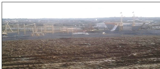
As the site is on elevated ground, there are great views of Ferrybank and Waterford City in the background.
