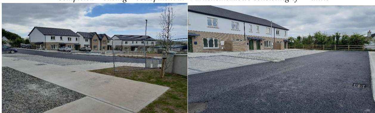
Housing Development at Abbeymount, Ferrybank near completion consisting of 16 units
