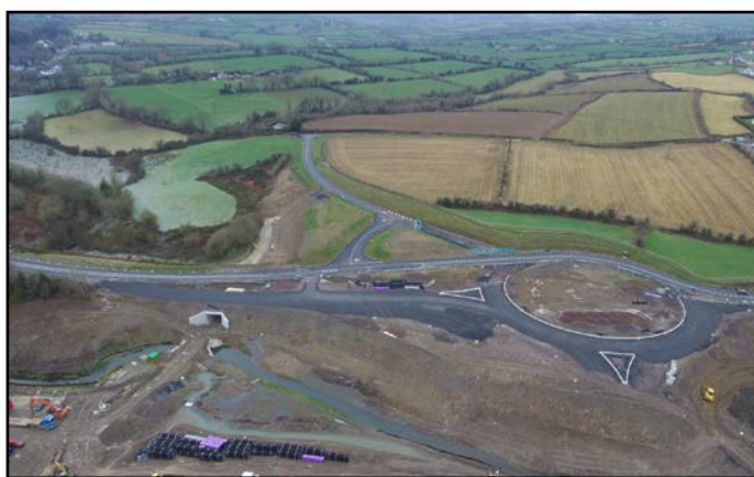
Works at Glenmore Roundabout and road underpass
