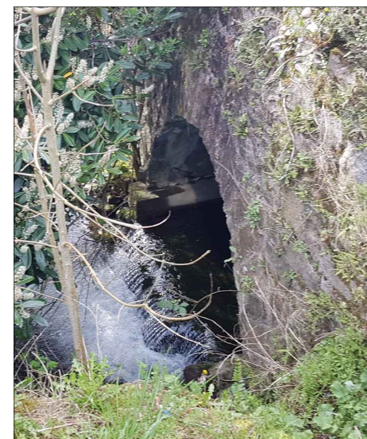
EXISTING OUTLET DROP TO BE REMOVED
