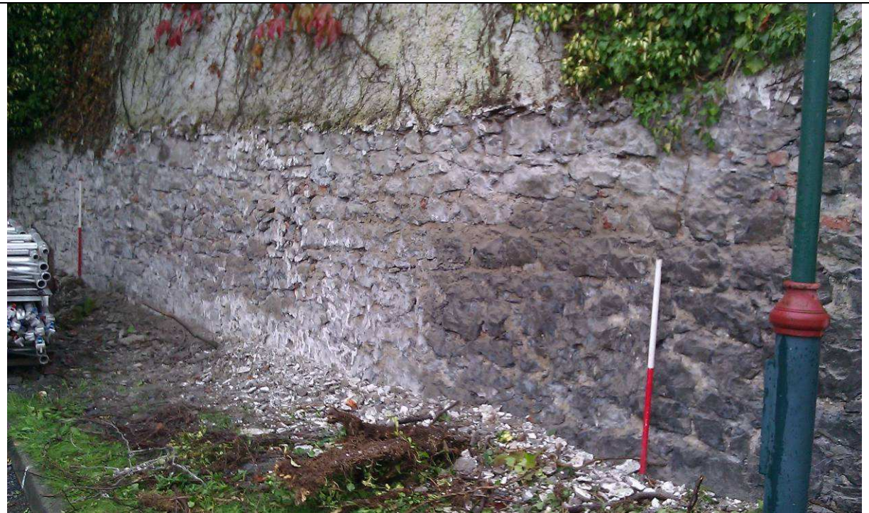
Plate 1: View of masonry wall C01 with pebble-dash removed, from Collegepark townland looking southwest.
