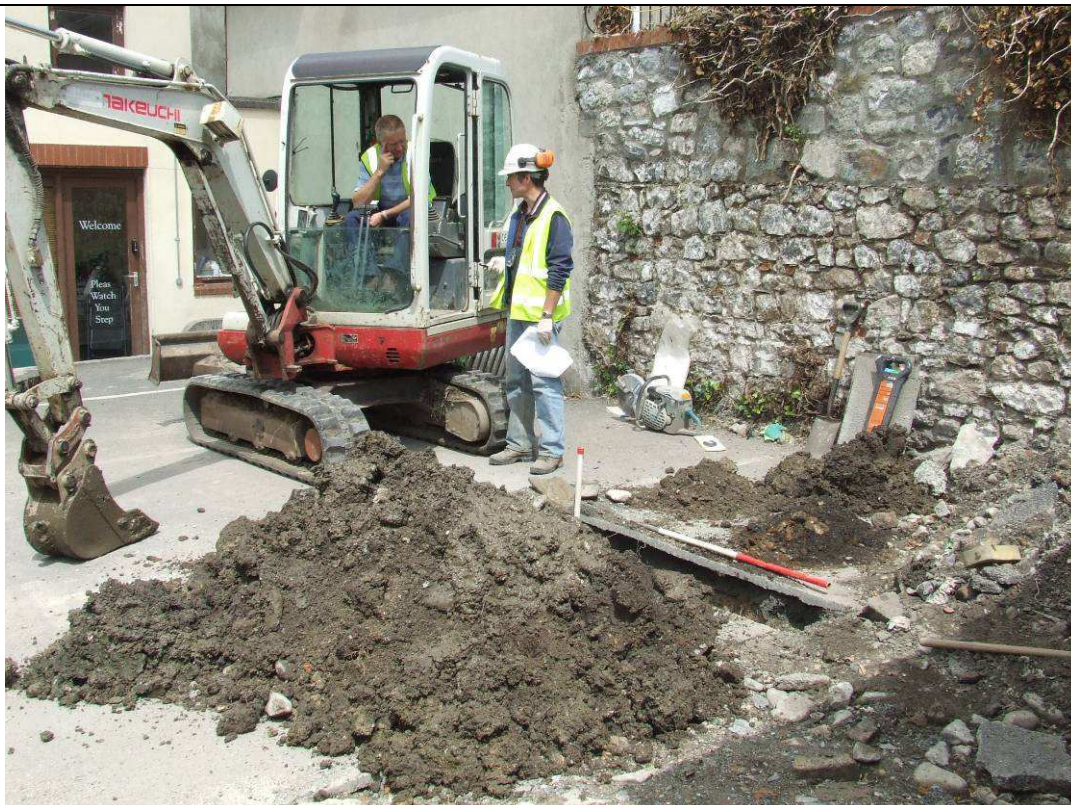
Plate 21: Trial Pit 2, under excavation, looking northwest.
