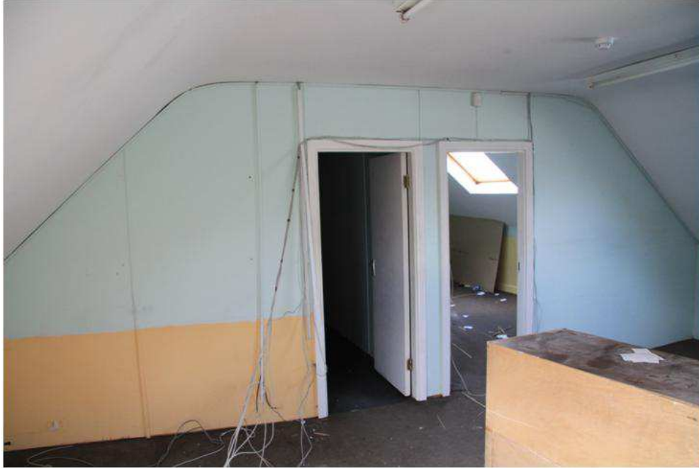
Plate 37: Doors to adjacent rooms in attic area
