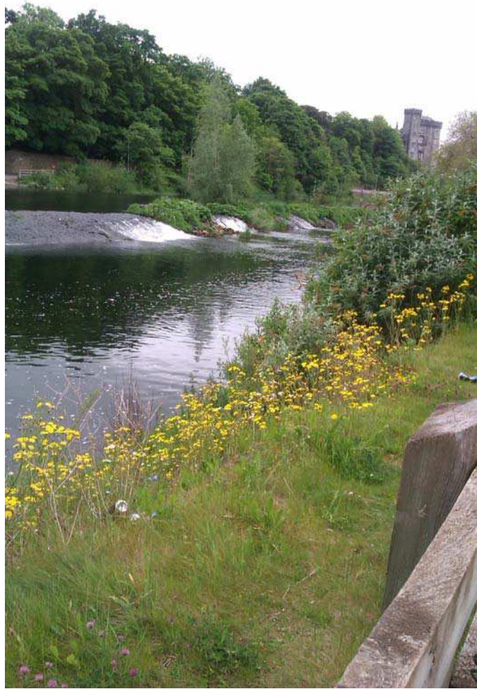
Photograph 5: Weir in River Nore by Site
