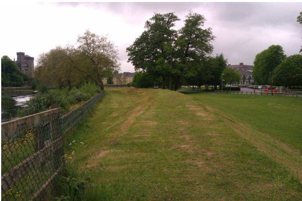
Photograph 3 & 4: Embankment on the Site
