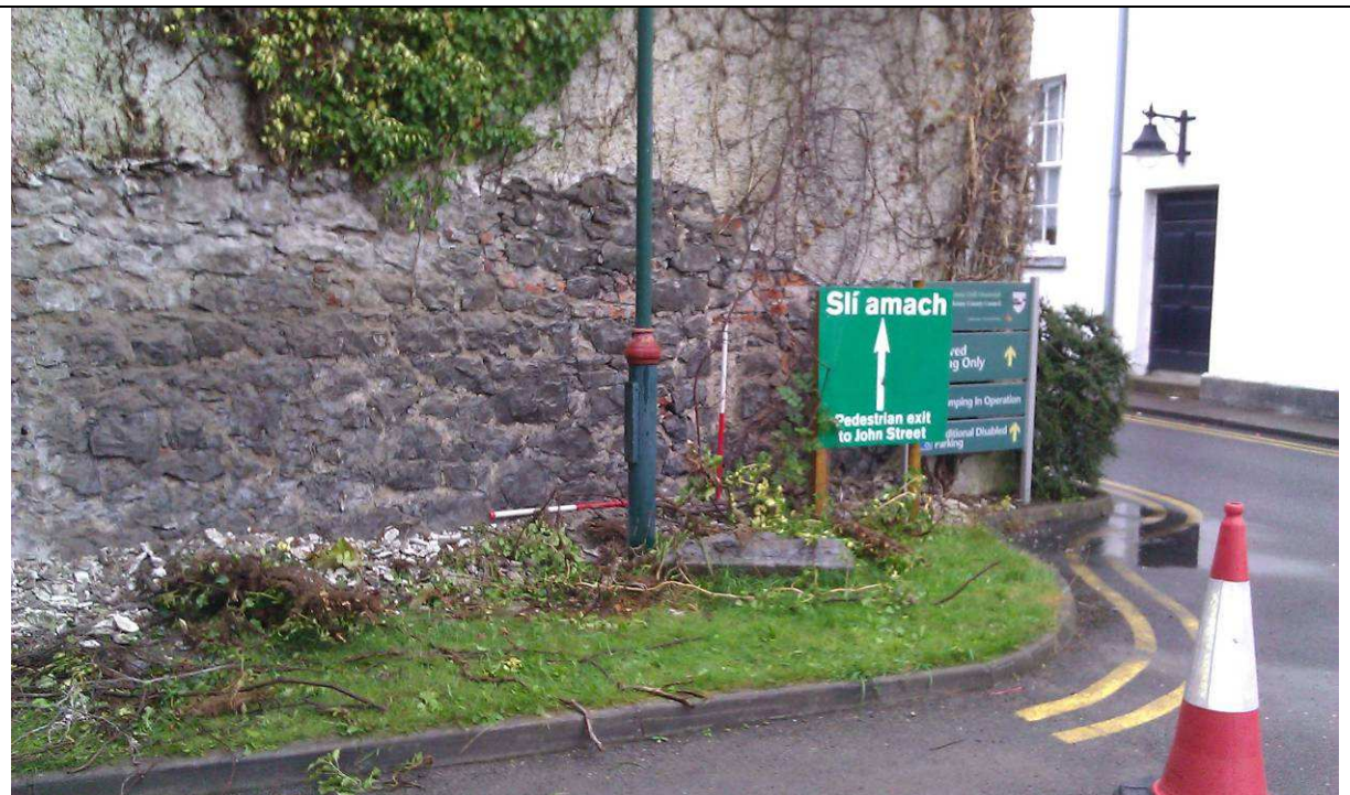
Plate 2: View of masonry wall C01 with pebble-dash removed, from Collegepark townland looking northwest.
