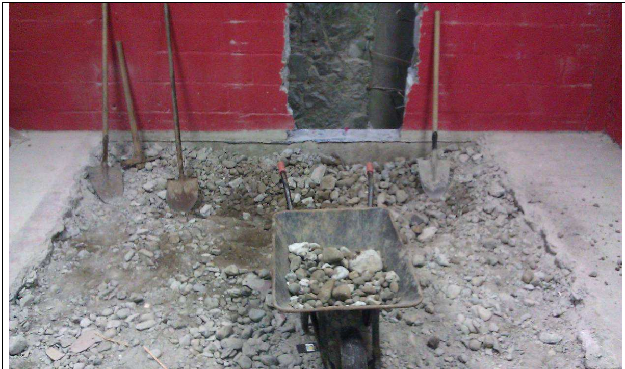
Plate 5: Trench VII showing initial removal of concrete floor and new opening in block wall. Looking southeast.
