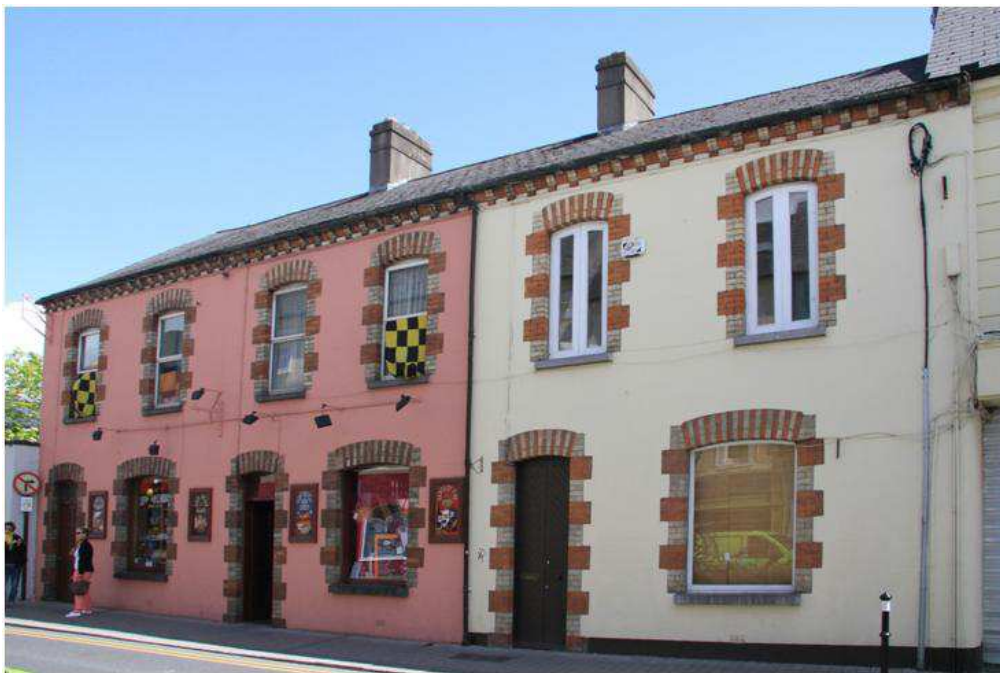
Figure 7: 73, 74 and 75 John Street Lower
