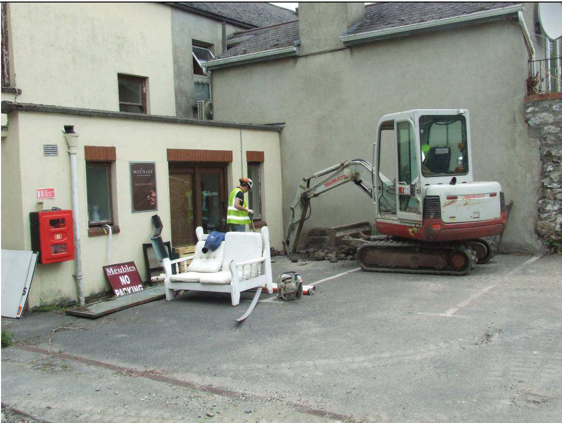
Plate 20: Trial Pit 1, under excavation, looking northwest.
