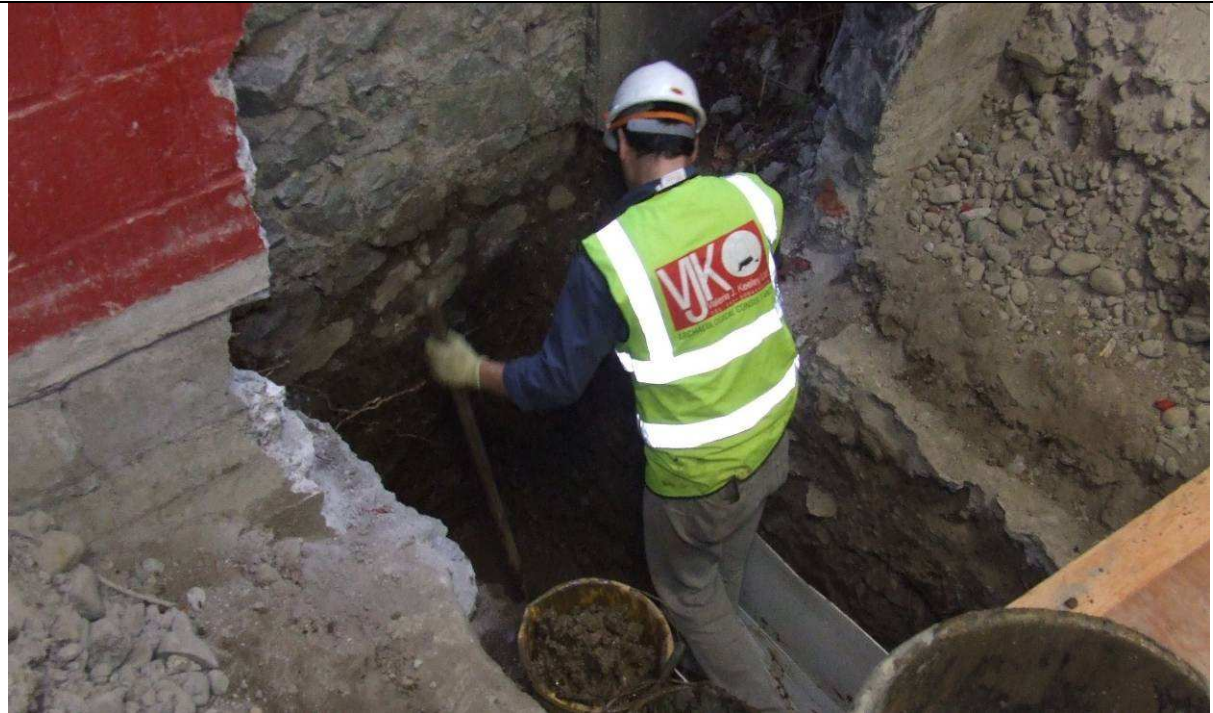
Plate 7: Trench VII following removal of 2 nd floor and concrete ring-beam under block wall C60. Looking south.
