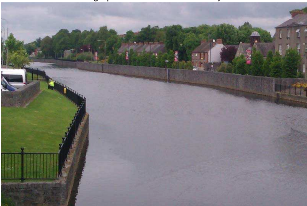
Photograph 6: Flood defences Upstream on the River Nore
