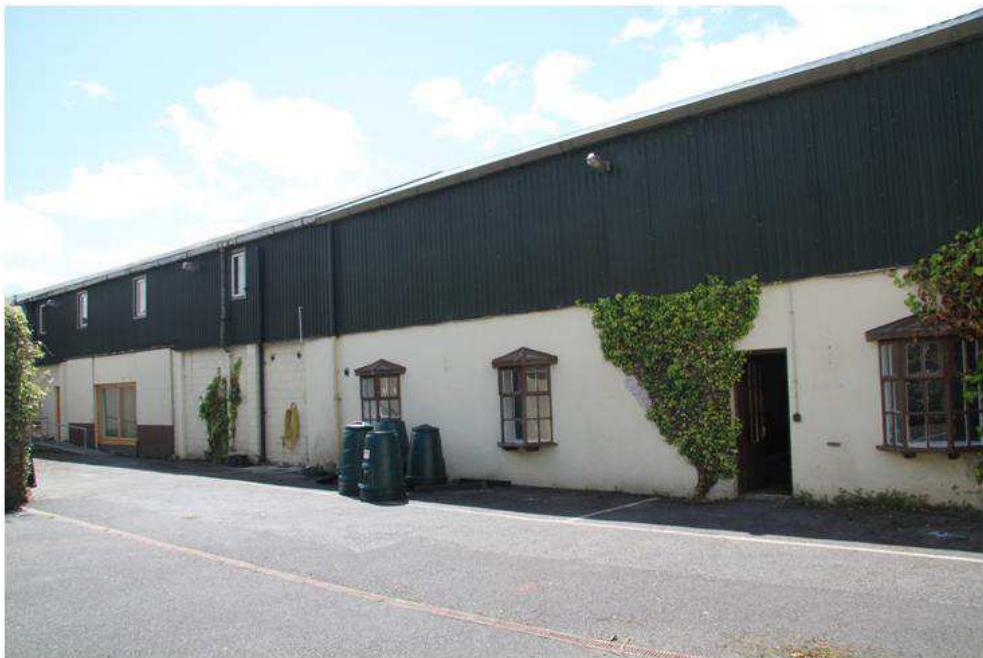
Plate 5: Return at rear of number 76
