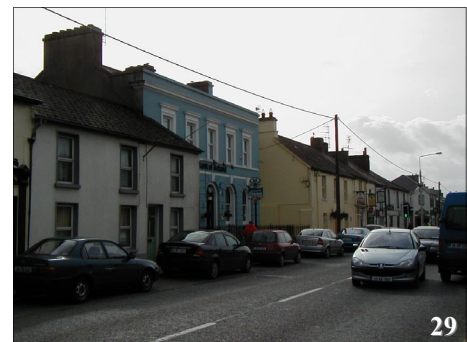
Photo 29: Traditionally set-backs in the building line were generally only reserved for important civic buildings, or as in this case a bank building.
