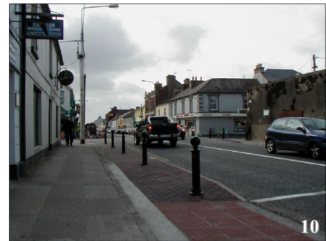
Photo 10: Example of pavement improvements that have occurred in the vicinity of Mill Street/New Line junction.
