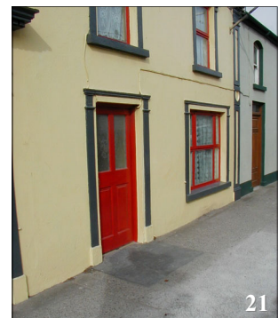
Photos 20 & 21: Attractive detailing around windows and door - note pseudo hood mouldings around bottom building. Both doorways have limestone flagstones on pavement entrance.
