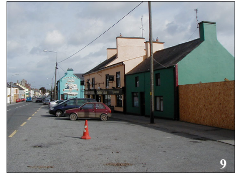
Photo 9: Example of streetscape between The Goul tributary and R689 junction where the building line gently curves giving way to significant space that could be considered for environmental improvements in the form of broader pavement, landscaping, treeplanting and car parking bays delineated by new surface materials and kerbing.
