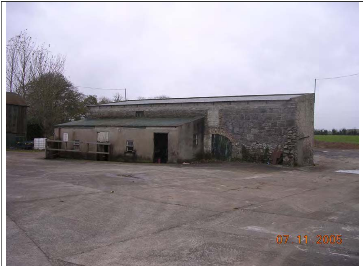
Plate 21. Looking west at AH6
