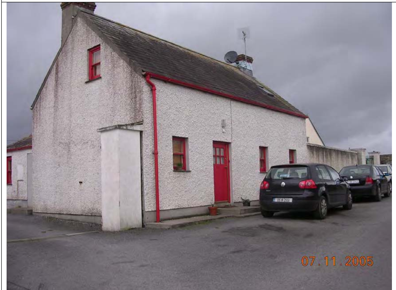
Plate 18. Looking northwest at AH4
