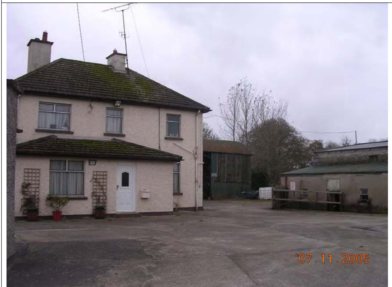
Plate 22. Looking south at AH6
