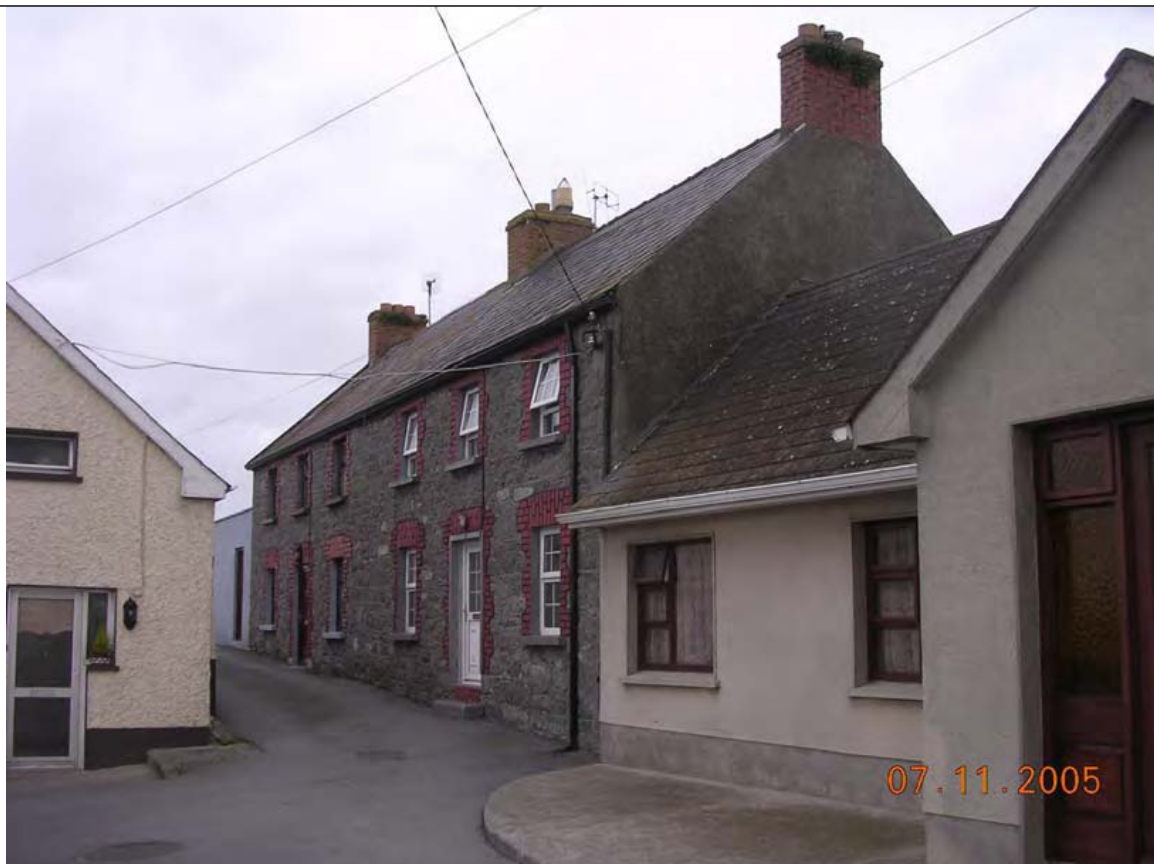
Plate 14. Two- story houses, facade of limestone to rough courses, gables rendered, brick window surrounds, brick chimney stacks. (AH2).
