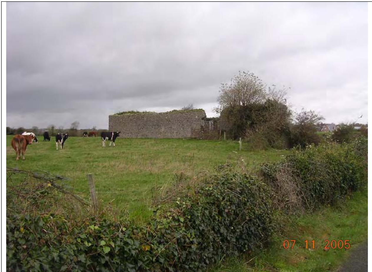
Plate 15. Looking north at AH3
