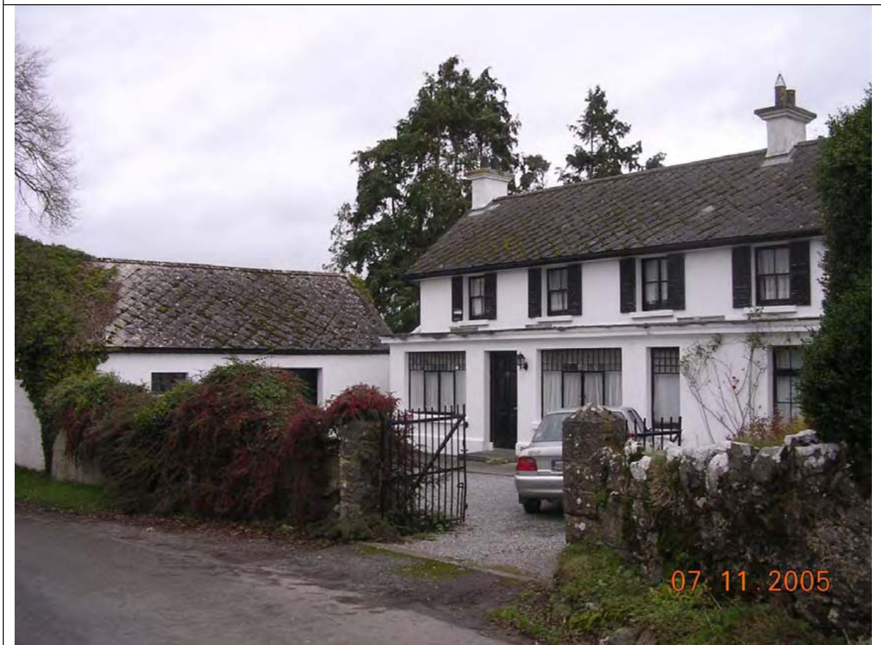
Plate 20. Looking north at AH5
