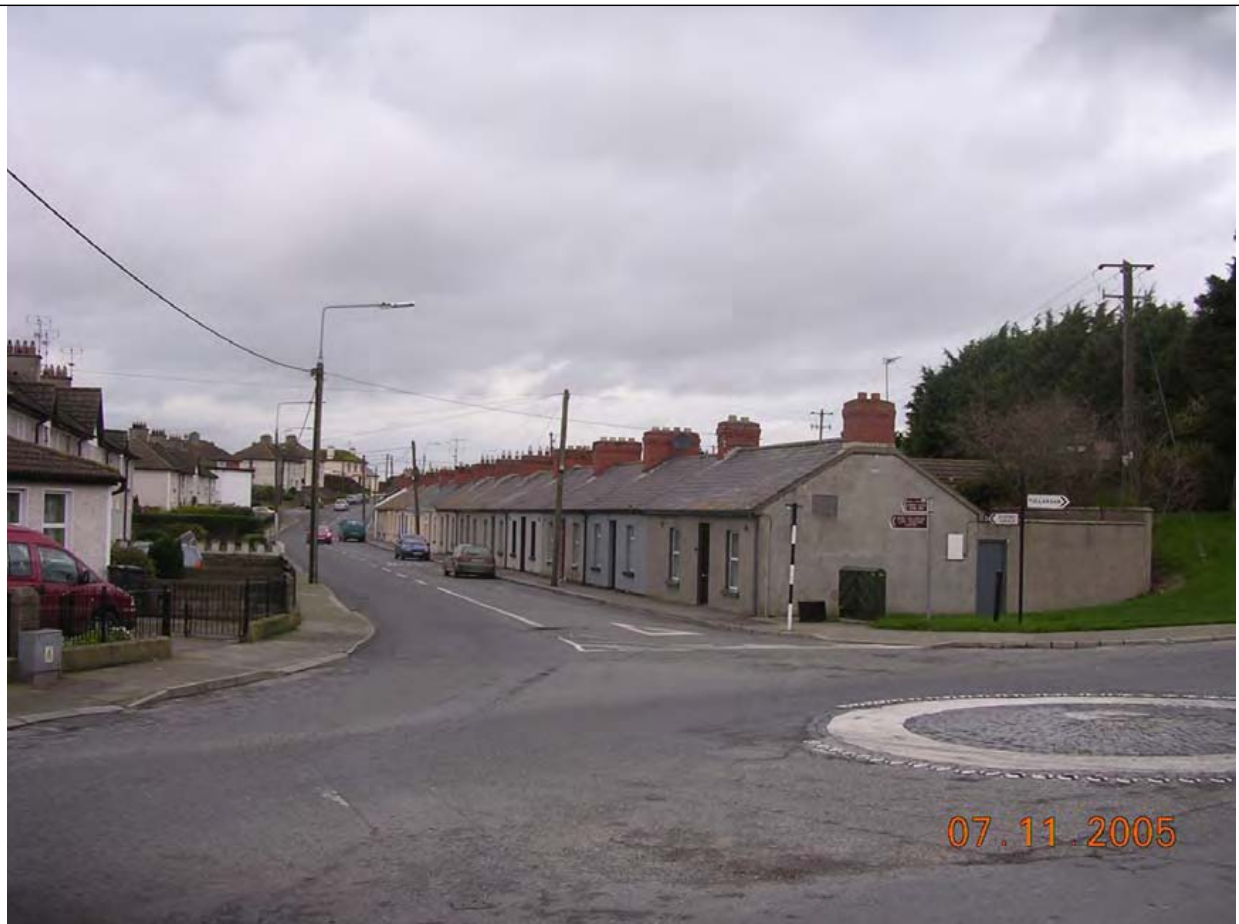
Plate 13. Terrace of one storey houses at the Butts, houses present at this location on 1 st ed. Current cottages 1910-1930 (AH1)
