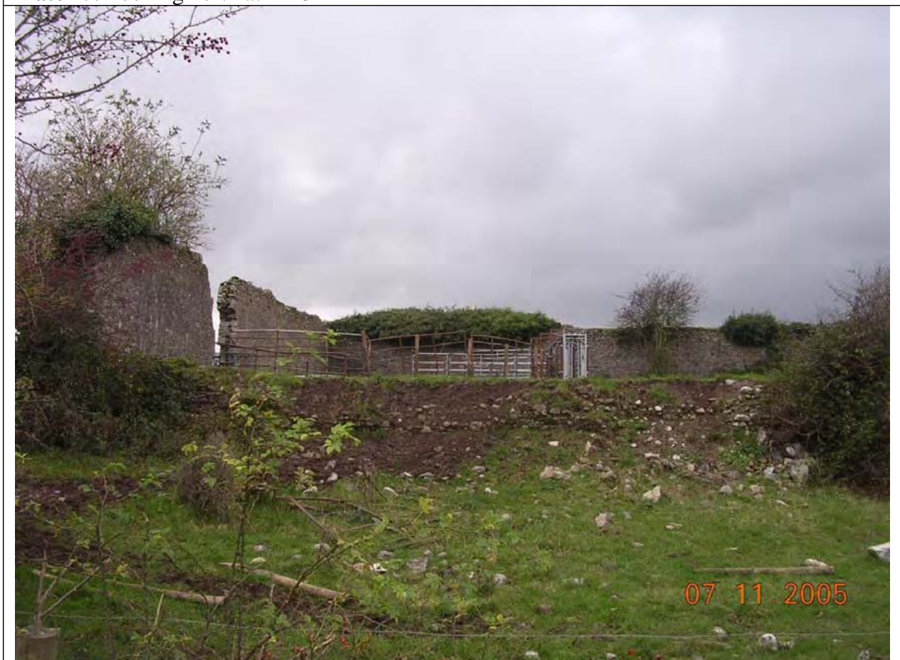
Plate 16. Looking west at AH3
