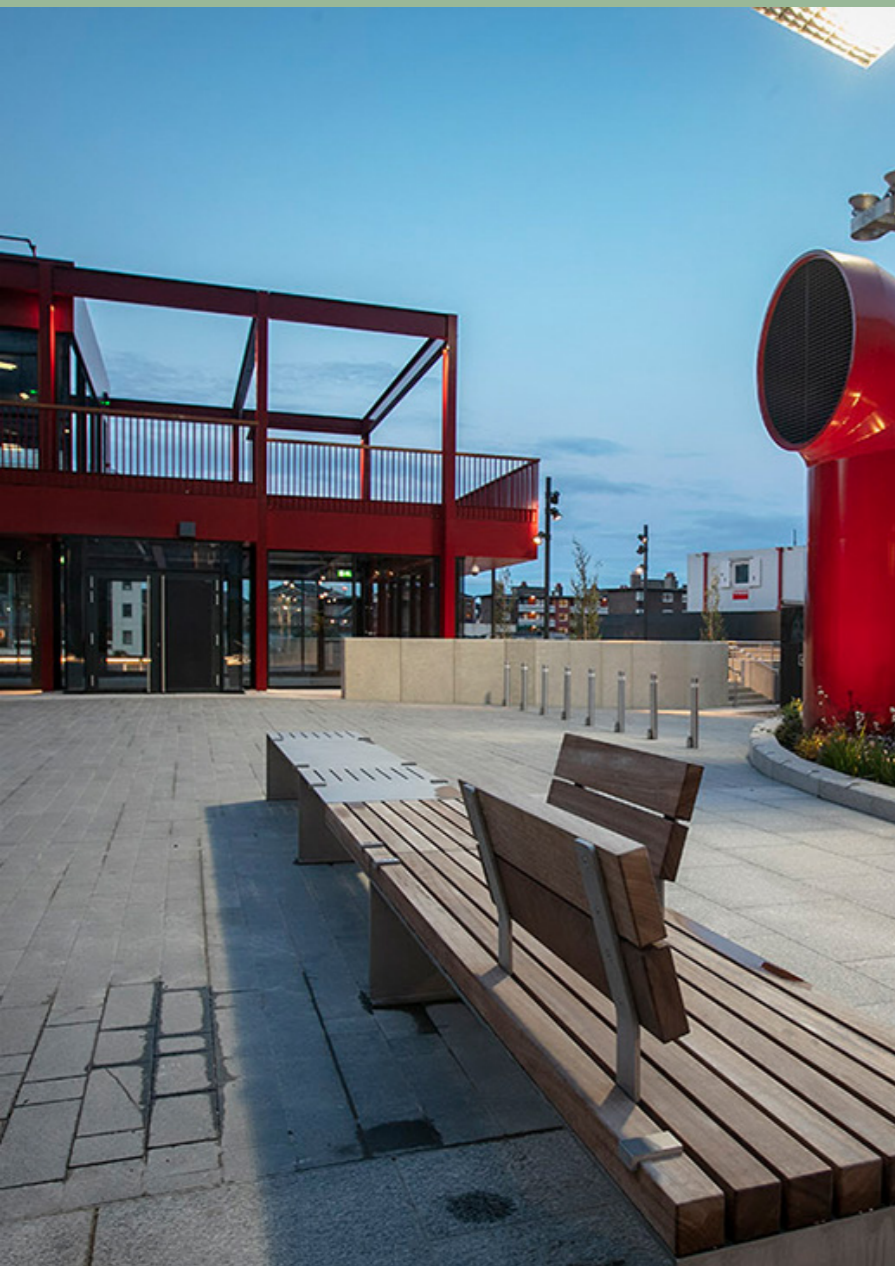
A new Ladies's Market/ Civic space on the river; the pumphouse will recede with appropriate screening, focusing on the pedestrian experience and journey.
