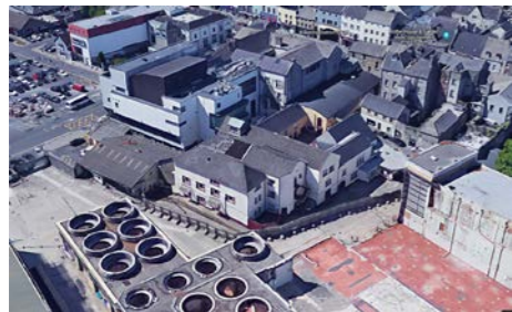
The Engineers' Block at The Smithwicks Experience
