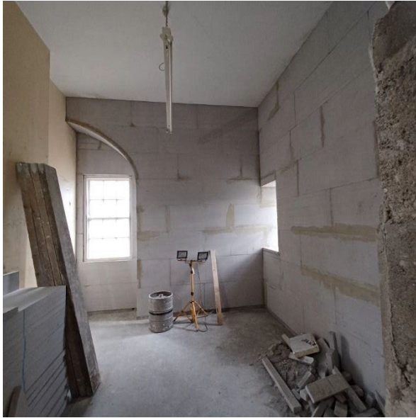
Fig.7 – Garda Station Back Office 2024 – Calsitherm Insulation
