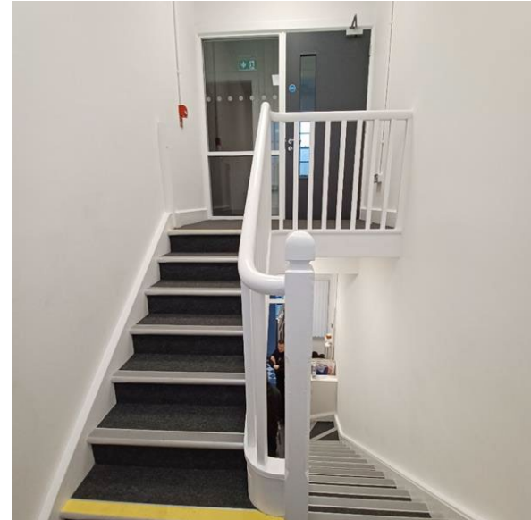
Fig.18 – Remote Hub Stairwell 2024
