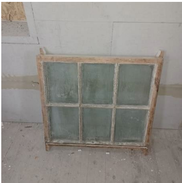
Fig.29 – Existing Window Repairs
