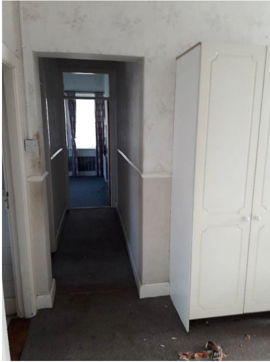
Fig.19 – Remote Hub 1 st Floor Landing 2023
