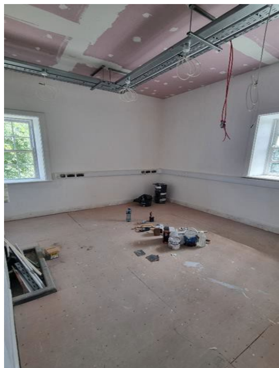
Fig.30 – First floor overlay -fire upgrade
