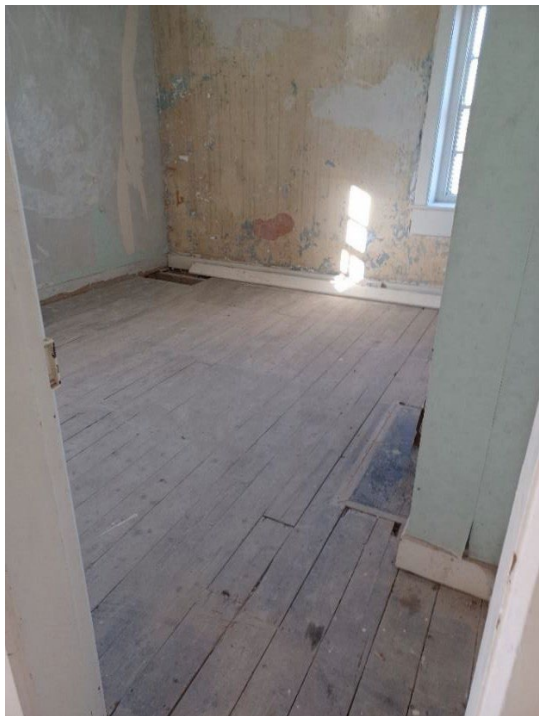
Fig.21 – Remote Hub 1 st Floor Office 2023
