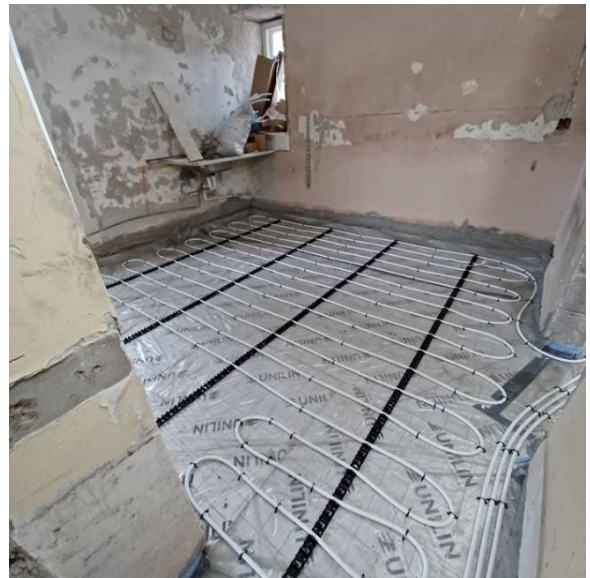
Fig.6 – Garda Station Back Office 2023 – Underfloor insulation and heating
