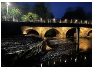
New Pedestrian Bridge, Castlecomer
