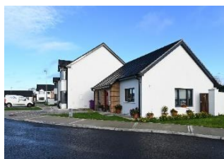
Station Avenue, Ballyragget.
