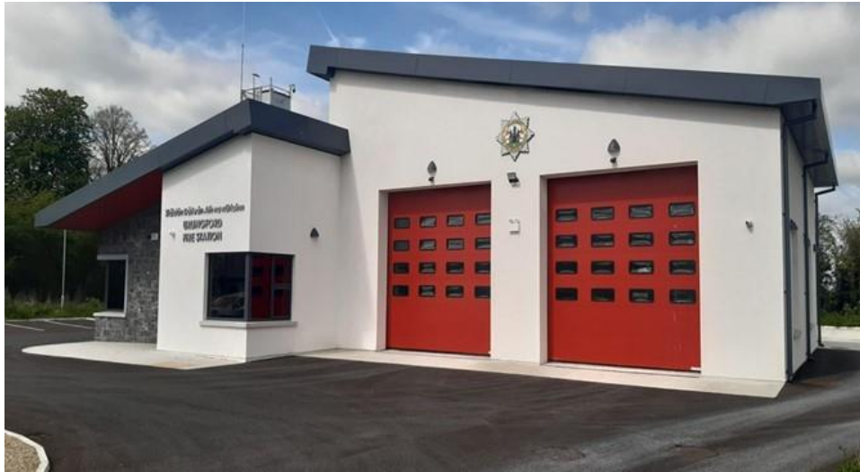
Fire Station, Urlingford
