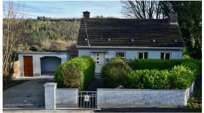
Former Health Centre Windgap - refurbished to 1 bed home. Completed 2020 by KCC
