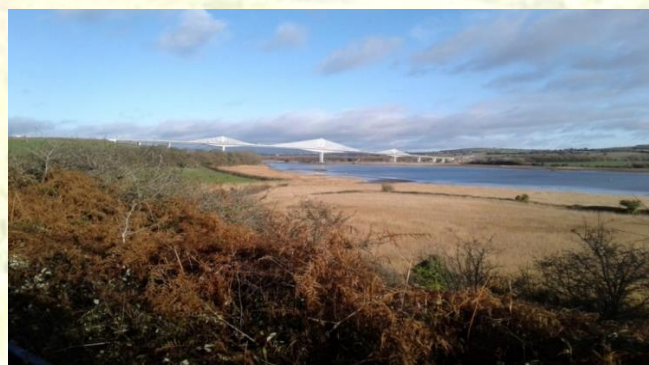
View of the Rose Fitzgerald Kennedy Bridge from the railway line at Carrickcloney
