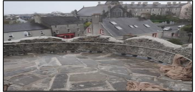
View from the newly repaired roof at Talbot's Tower
