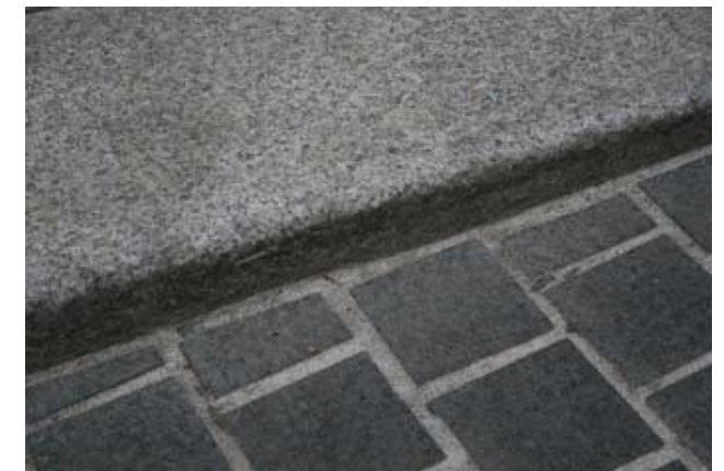
Detailing the footpath
