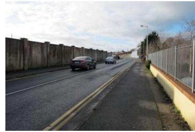
'Dead' frontage at Nowlan Park
