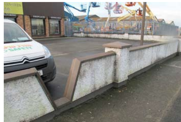
Pedestrian wall feature
