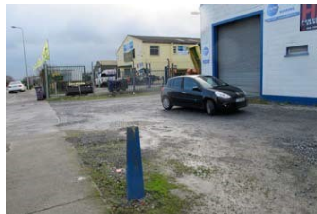
Poor quality frontage
