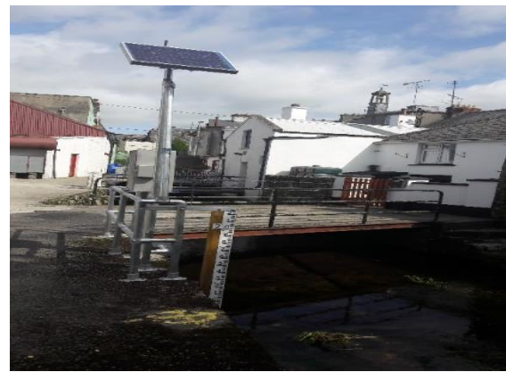
New Water Level Gauge – Turf Market
